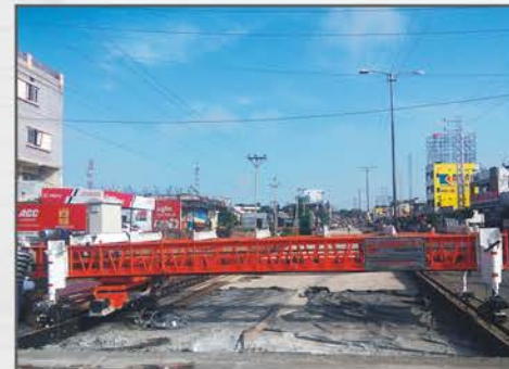
Concrete Road Paver (Fix Form Paver)
