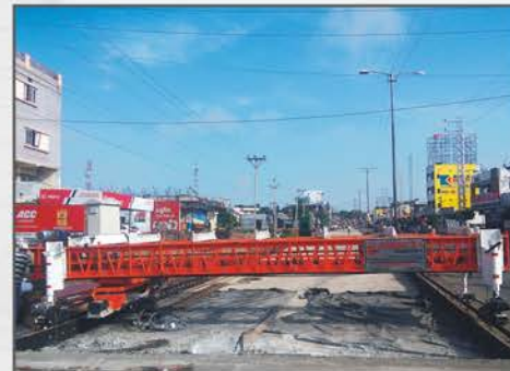
Concrete Road Paver (Fix Form Paver)
